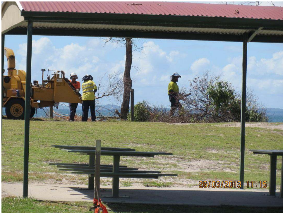
Clearing the last remaining vegetation - Woorim foreshore, South Boyd Street.
