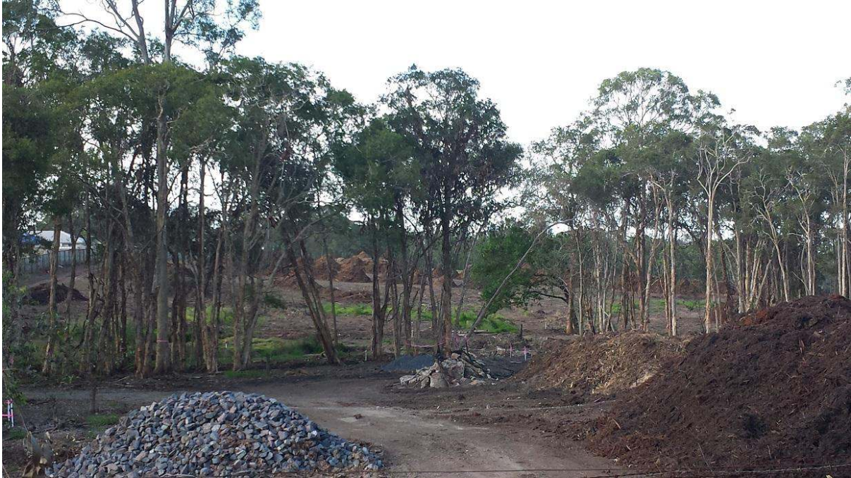
Alma Road Dakabin. Piles of woodchip foreground and background. Loss of habitat and wildlife.
