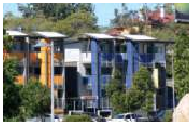
Affordable apartments in the suburbs
