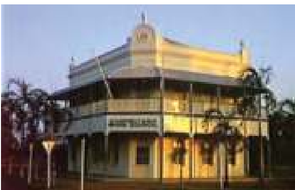
Landmark buildings as key parts of centres
